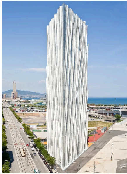
Figura 25. Torre Diagonal One
